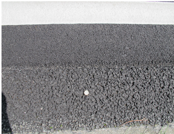
Figure 4: Two layer porous asphalt
