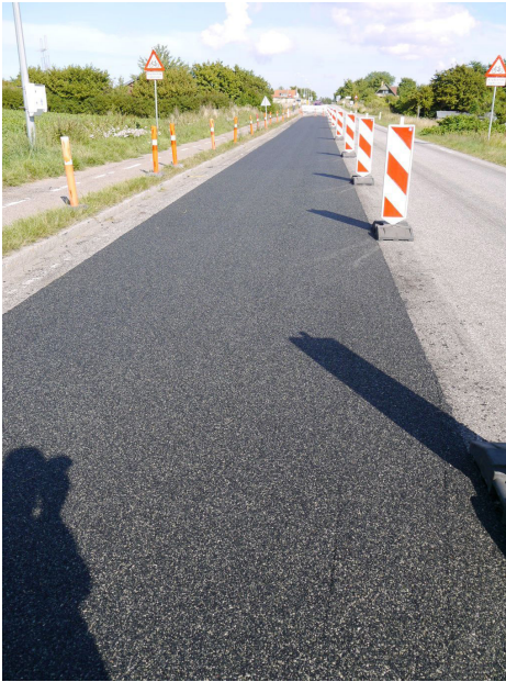
Figure 6: Test section with poroelastic road surface in Kalvehave (Denmark)
